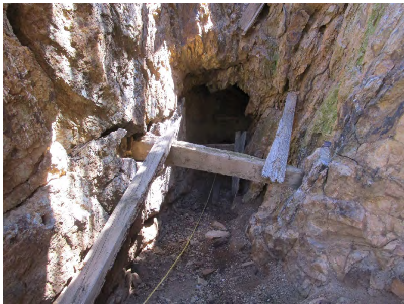
Figure 20. Portal to the 25 ft level McNary Mine-photo by Morris.
